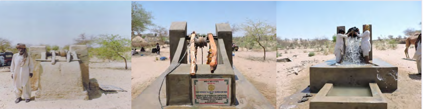
Before (left) and after (centre and right)
